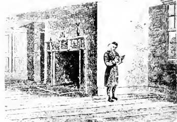
CHIMNEY OF BED-ROOM ON SECOND FLOOR.
